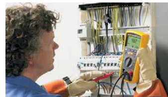
Insulation test at a distribution panel
