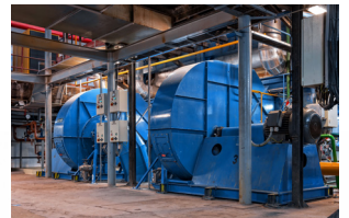
Noise and vibration
